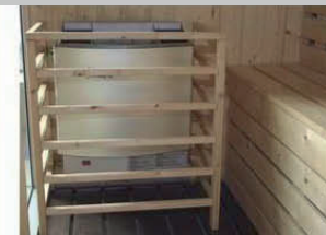
Wooden frame for protecting sauna heat generator
